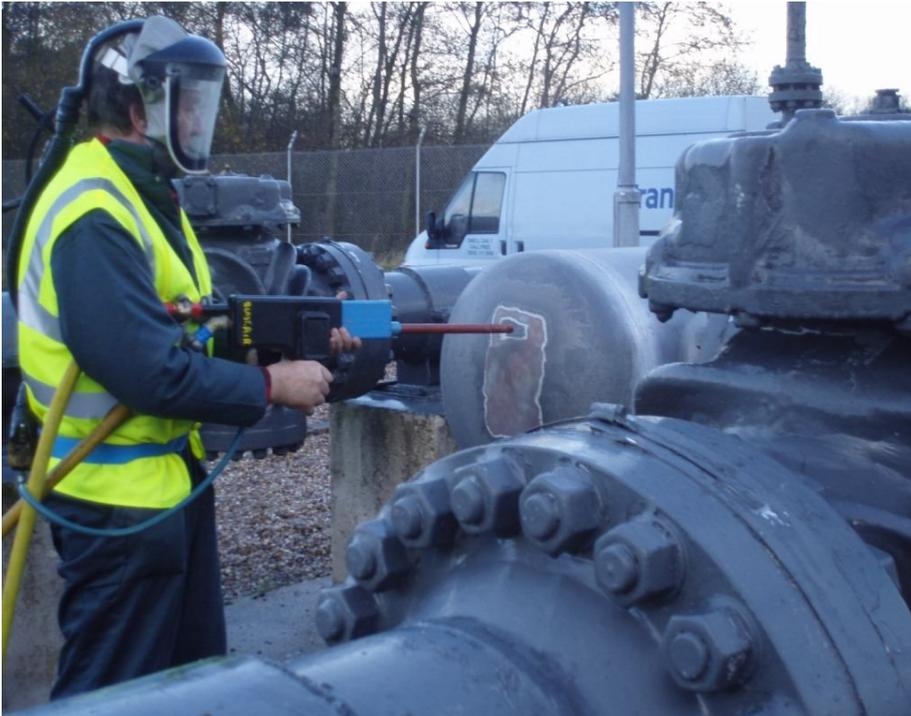
The second photograph shows the area of blasted steel and the edges which are naturally feathered by the crushed glass. The finish was sufficiently clean of all debris & paint to carry out NDT inspection if required
