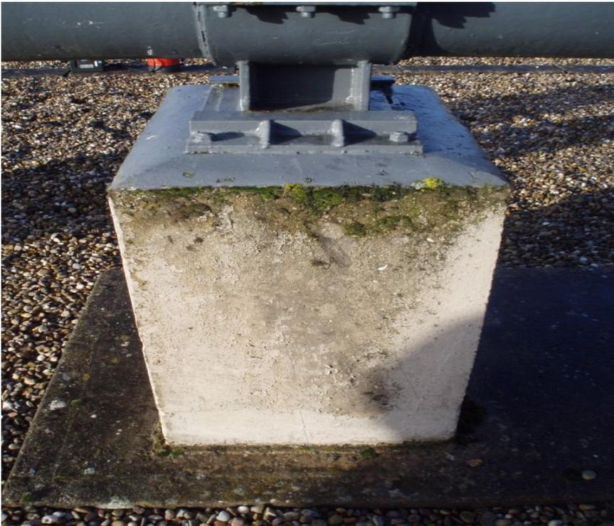
Photo 4 shows the same pillar after blasting using DORIS with fine glass & water spray for approx 3 minutes. All signs of algae & growth have been removed to allow paint to be applied when dried. There were no visible signs of contaminated spent grit to clean up.
